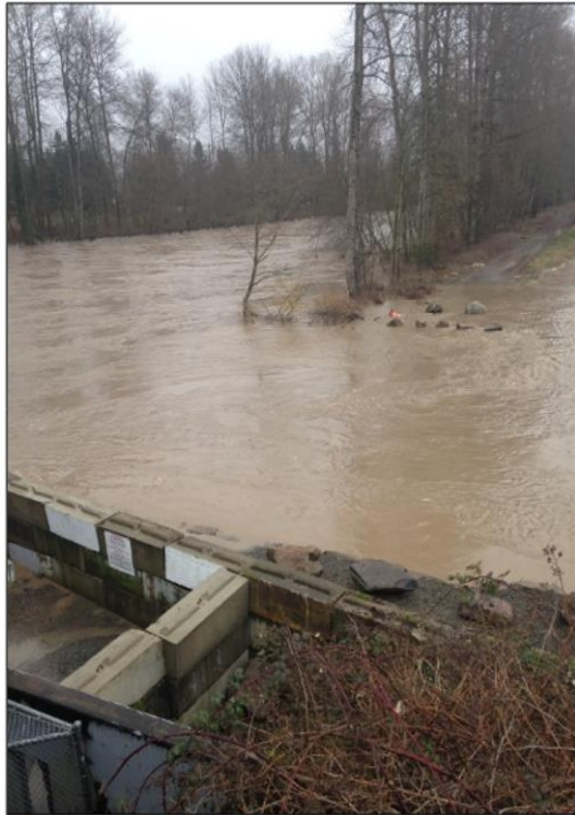
Figure 4-22. SVC 2020 photo 9, taken from the north, showing floodwater covering the entire outfall facility in February 2020.
